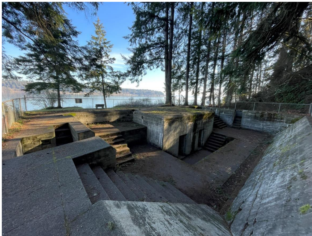
What remains of the Battery Mitchell, looking out across Rich Passage to Fort Ward and Bean Point.
