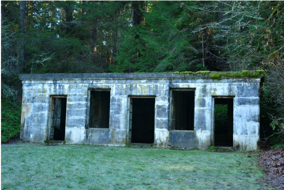
The Casemate where operators would have been sought shelter when mines were detonated.
