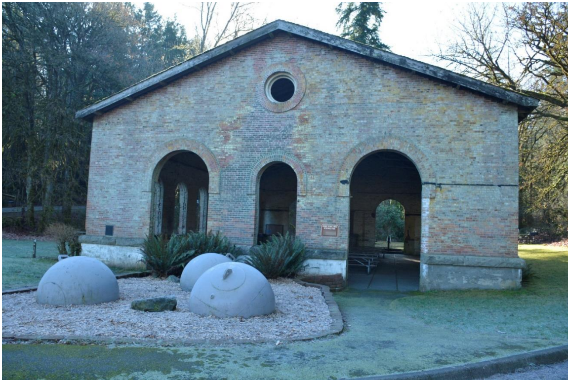
The front of the Torpedo House, with some of the underwater mines that would have been filled with explosive and networked together by electrical cables.
