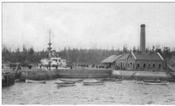
"Monterey" gunboat in Port Orchard dry dock. Transcribed from back of photograph: "The Monterey in dry dock... They put the boats in the dock, then pump out the water to paint or clean the bottom which gets covered with barnacles, little muscle shell, sea Courtesy The Seattle Public Library Special Collections Online (spl_lj_063)
