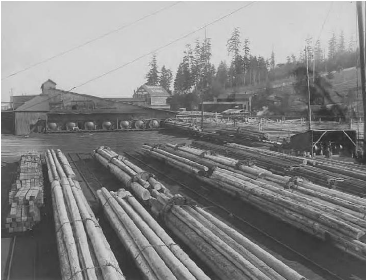
Railroad cars with logs and retort at Pacific Creosoting Company, Eagle Harbor, approx.. 1909. Property of University of Washington Libraries, Special Collections.
